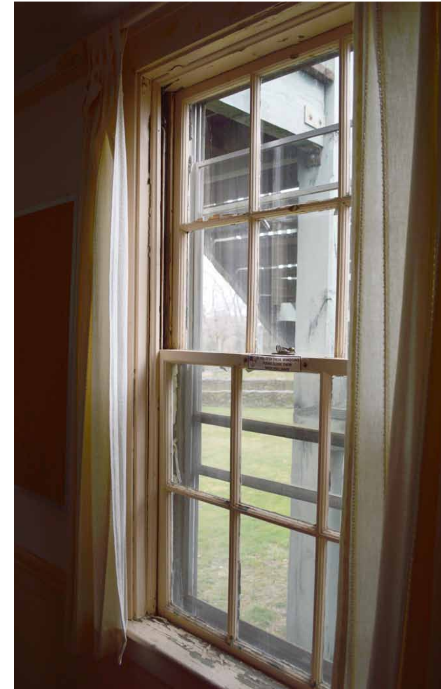
The windows are in varying states of disrepair. Many require repainting and replacement of rotting sills.
