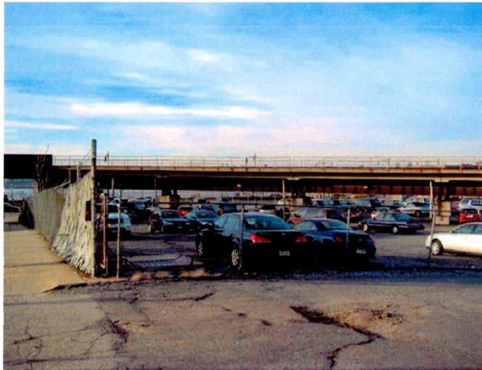
Photograph E: View From East
