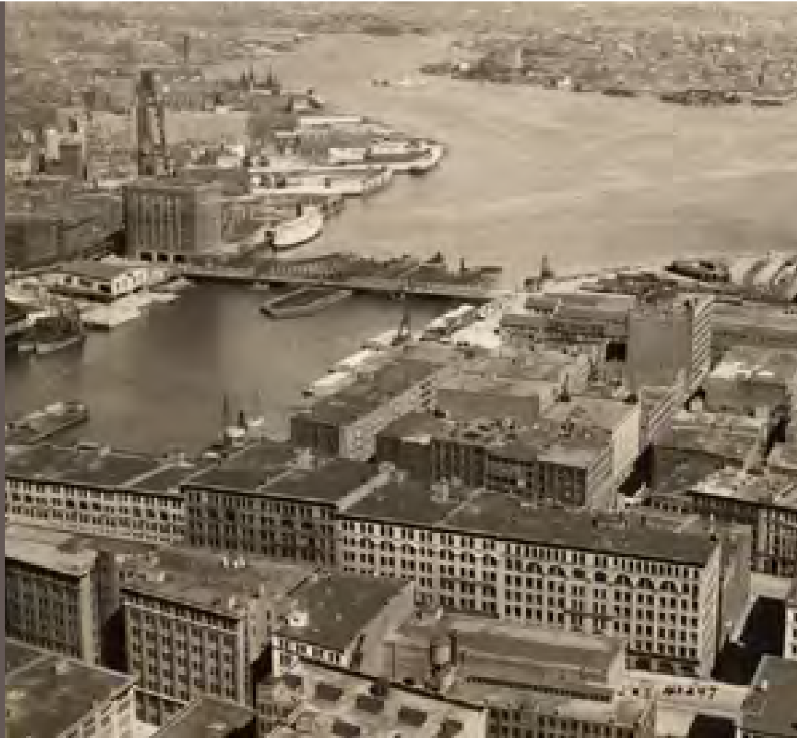
Areal view of the Fort Point Channel District and the Channel itself circa 1900.
