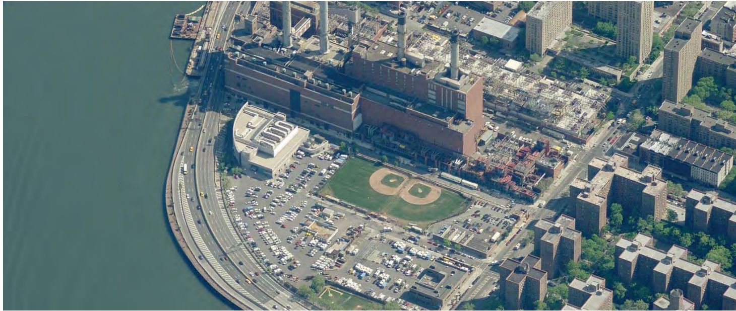
Aerial looking south. Notice the large power plant adjacent to the site.
