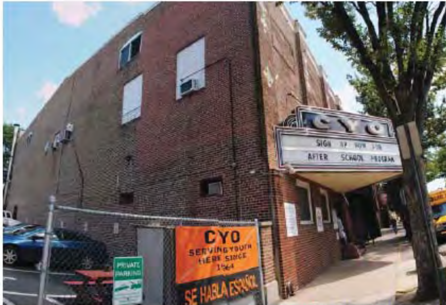
Side entrance to the CYO building in front of the parking lot.
