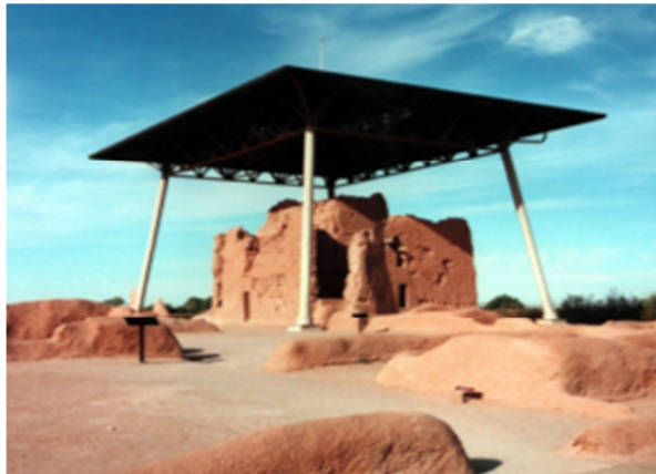
Figure 14 Casa Grande New Roof Structure, 2009, nps.gov
