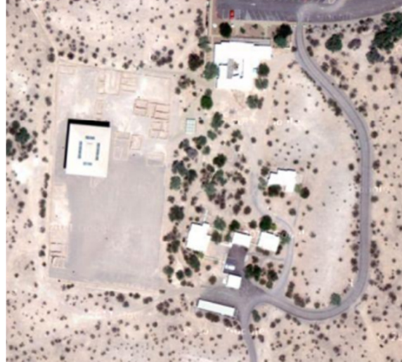
Figure 9 Casa Grande National Monument, aerial view, maps.google.com
