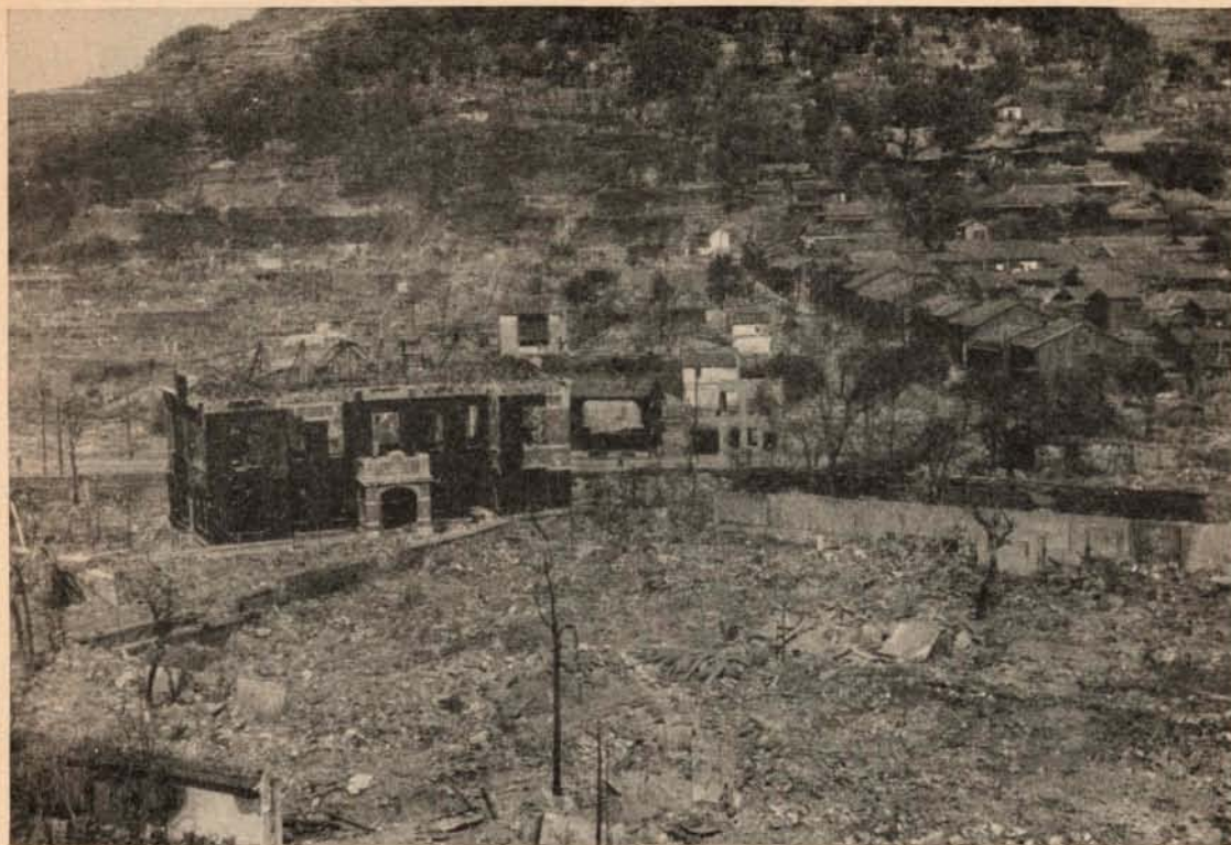
FIRE FRINGE. 8,200 feet from ground zero at Nagasaki, the old police station was completely gutted by fire. Hills protected houses on the right from blast, and fire did not spread to them (Japanese photo).
