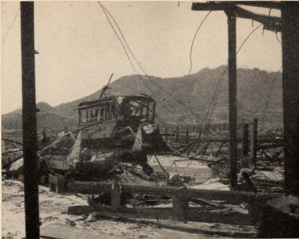
WRECKAGE IN NAGASAKI STREETCAR TERMINAL 1,500 feet north of ground zero. Streetcar in center was blown about 6 feet by the blast (Japanese photo).
