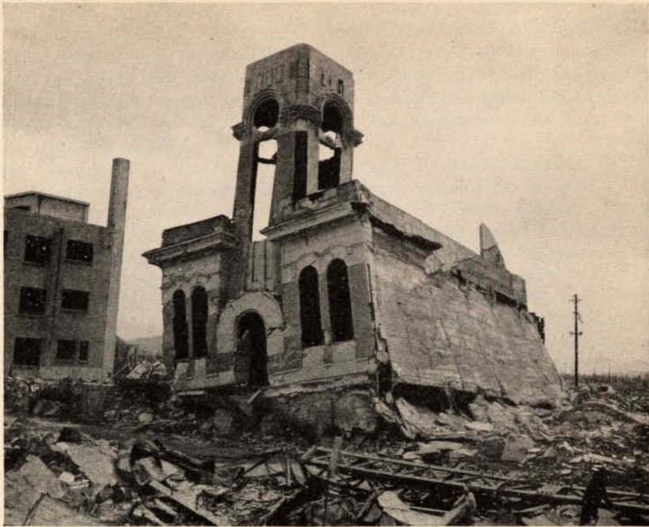
THIS STEEL FRAME BUILDING, 2,000 feet from ground zero at Hiroshima, had its first-story columns buckle away from the blast, dropping the second story to the ground. Combustibles were destroyed by fire.
