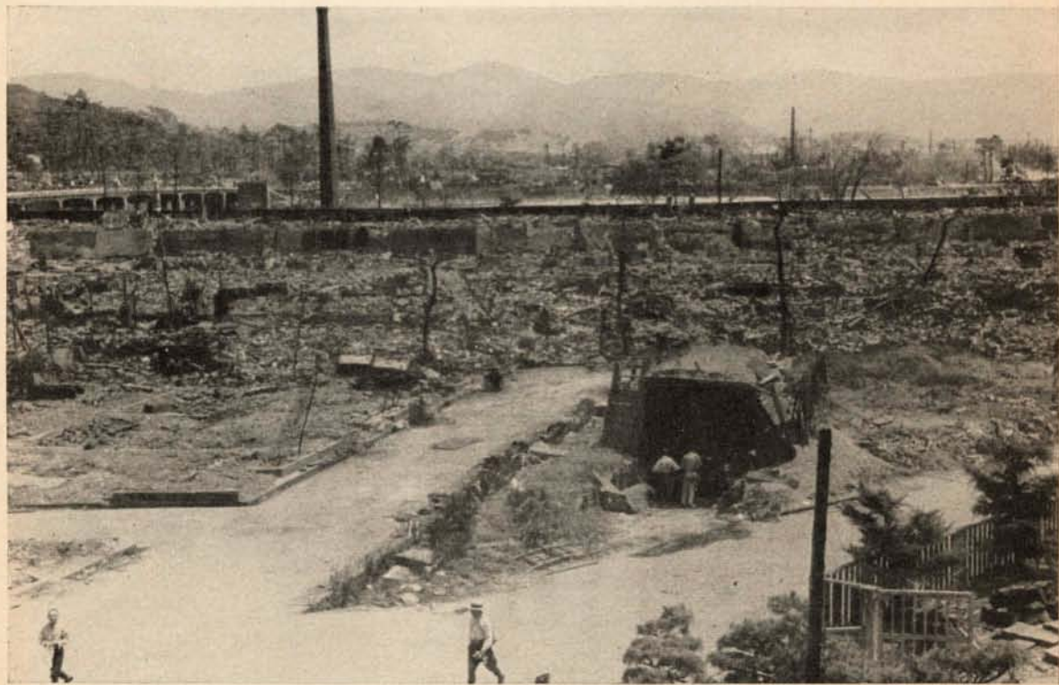
HIROSHIMA EARTH-AND-POLE AIR-RAID SHELTER. This simple shelter is undamaged by fire and blast 5,000 feet northeast of ground zero, though surrounding buildings have been destroyed (Japanese photo, 10 August 1945).
