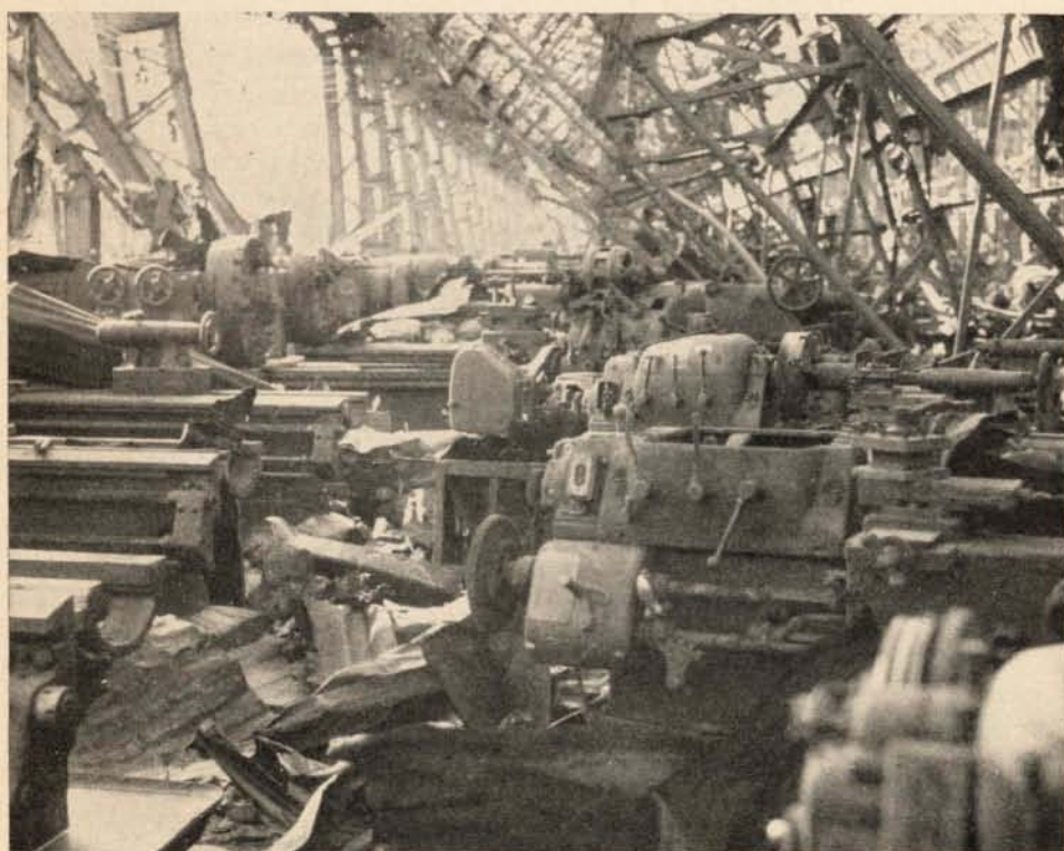
DAMAGE TO MACHINE TOOLS was usually indirect. At the Mitsubishi Steel and Arms Works, 4,200 feet from ground zero at Nagasaki, many closely packed machines escaped serious damage from collapsing roof trusses, but were exposed to the weather. Other machines were torn from their foundations by collapsing steel members.
