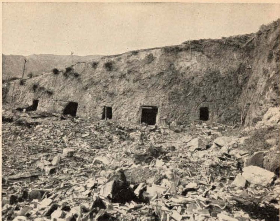
NAGASAKI SHELTERS. Tunnel shelters in the hillside, such as the ones pictured (very close to ground zero), protected the few occupants from blast, heat, and radiation.
