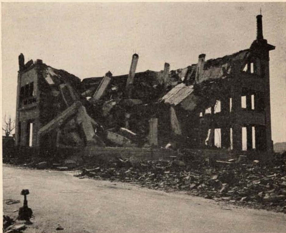
COLLAPSE OF REINFORCED CONCRETE BUILDING. Chugoku Coal Distribution Control Co., 700 feet from ground zero at Hiroshima.
