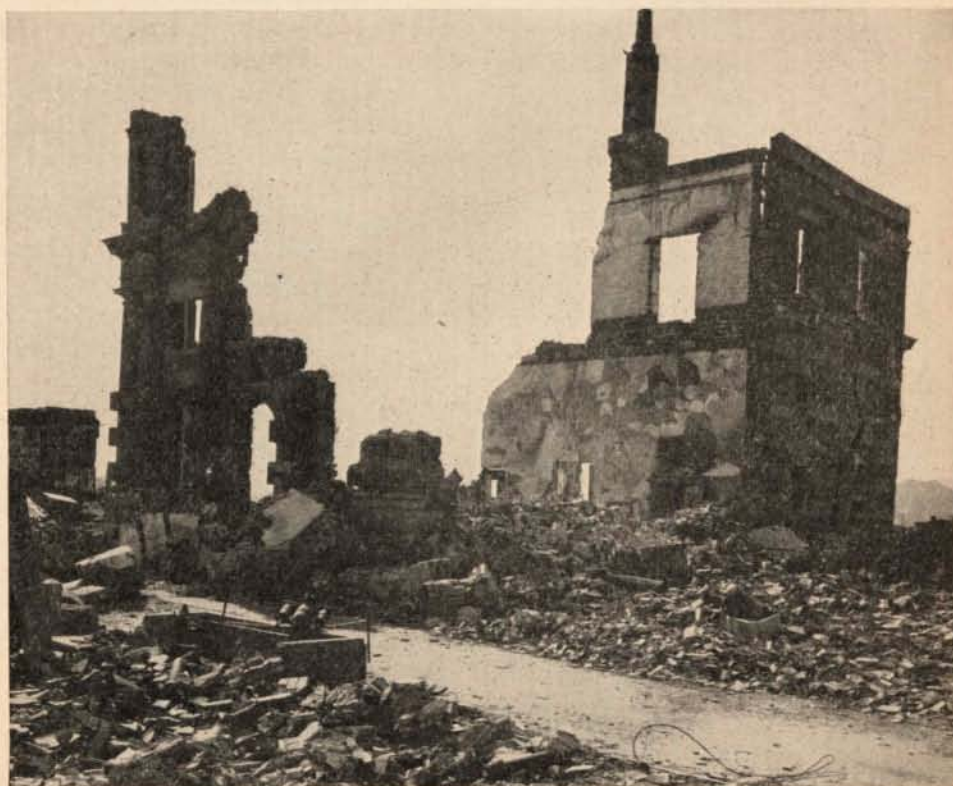
DESTRUCTION OF BUILDINGS WITH BRICK LOAD BEARING WALLS. Note how brick debris lies inside wall facing blast, at remains of a barracks at the Japanese Army Divisional Grounds, 4,200 feet from ground zero at Hiroshima. The Koa Fire Insurance Co., 1,300 feet from ground zero, is completely destroyed except for the heavy walls of the vault.
