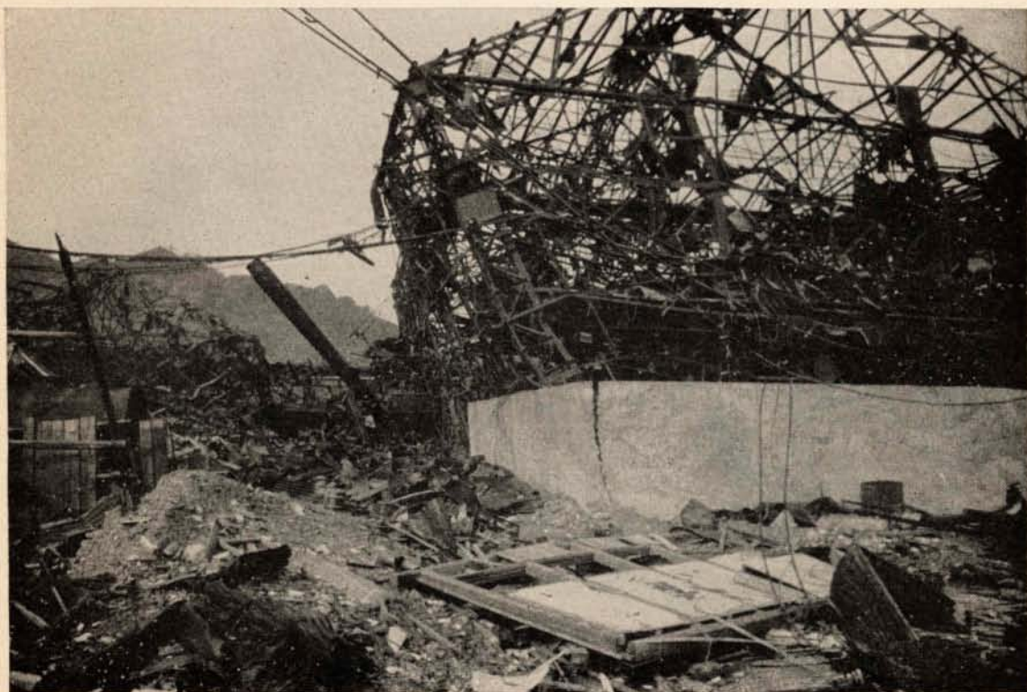
NAGASAKI. Steel-framed building about 4,000 feet south of ground zero in Mitsubishi Steel and Arms Works distorted to grotesque shape by blast of bomb.
