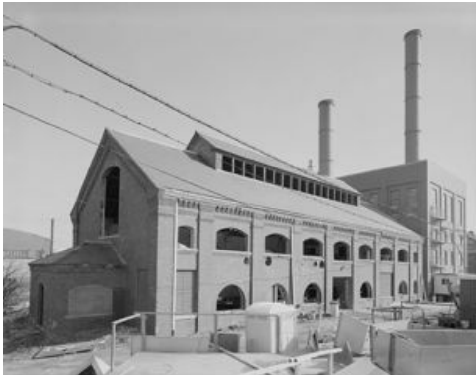
Chemical House at the Fields Point Wastewater Treatment Facility, March 1989. National Park Service.
