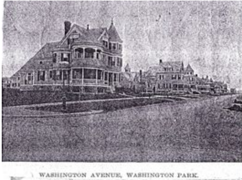
View of 305 Washington Avenue, looking northeast. The two-story porch on the southwest corner is no longer extant, but the three-story turret on the southeast corner still remains. Note 287 Washington Avenue in the background. Rhode Island Historical Society.
