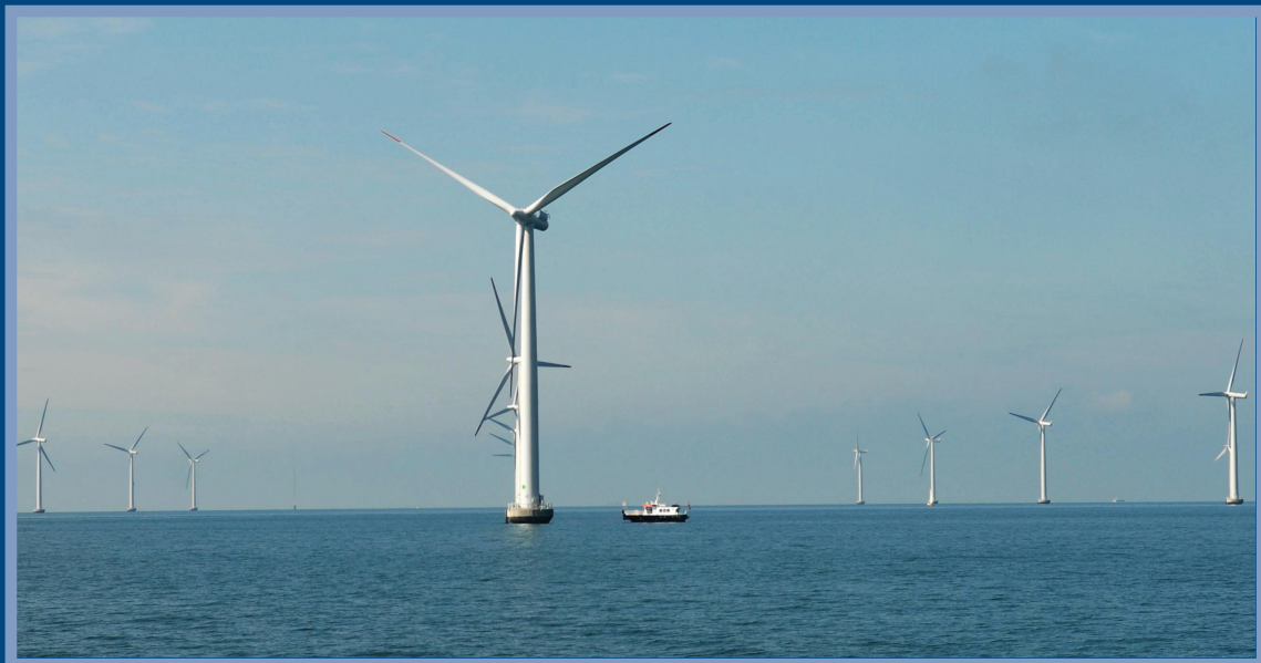
Photo courtesy of Bluewater Wind
