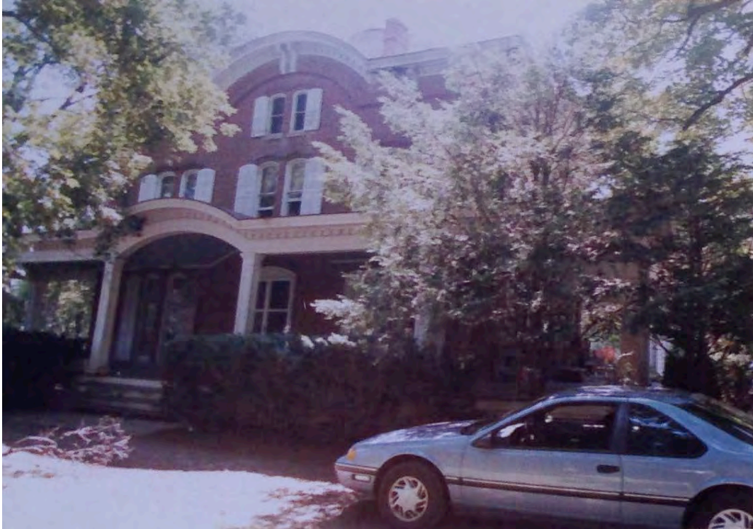
McCloughan Mansion circa 1989. East Elevation. Clinton Township Tax Assessor. July 29, 1989.
