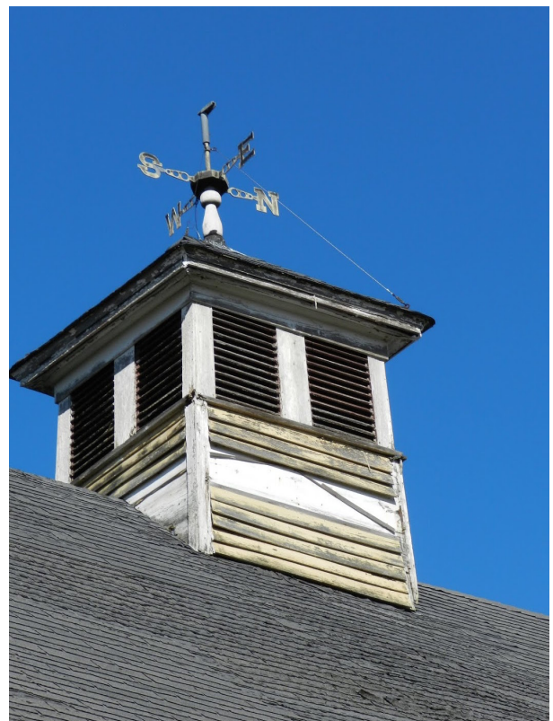
Figure 25.4: Cupola and Weathervane on roof
