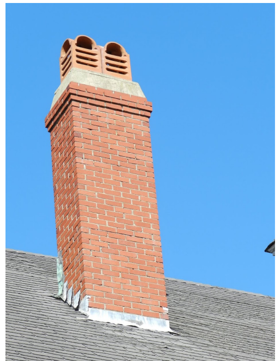
Figure 23.4: Chimney view at East elevation
