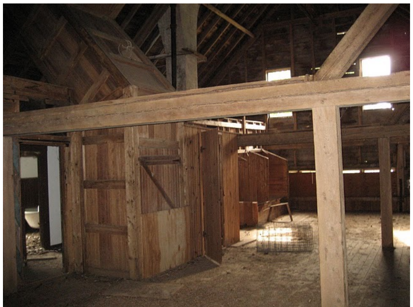
Figure 29.4: Interior Structural Beams
