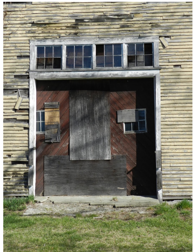
Figure 27.4: Door and Transom Window North Elevation
