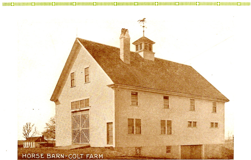
Figure 1.1: 1901 Historic Photograph of Stable
