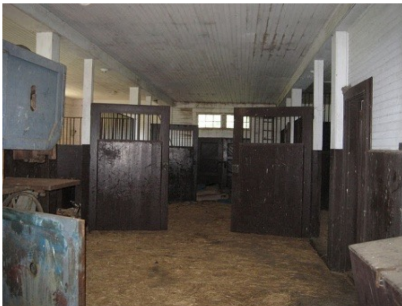
Figure 30.4: Interior doors and board and batten paneling
