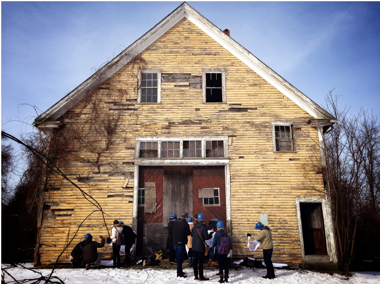
Figure 18.4: Existing condition of North elevation
