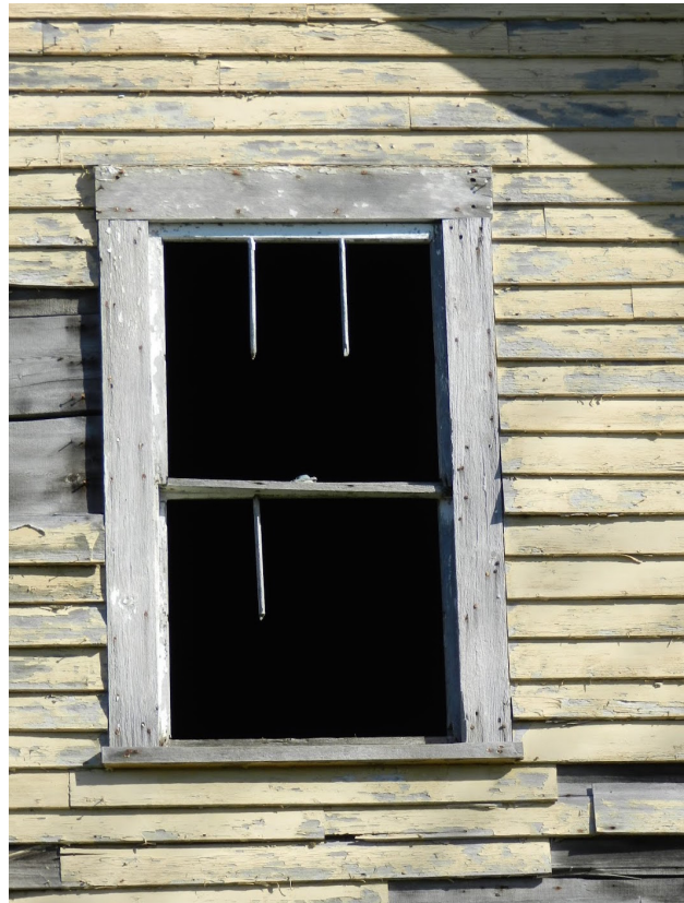
Figure 26.4: 6-over-6 Double Hung Window on North Elevation
