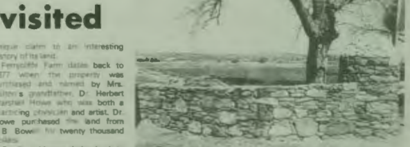
THE MAIN ENTRANCE. As it is seen today, was refurbished this spring in the same form as the original entrance looked like to Ferrycliffe Farm. MRS. FULTON has said that DR. FULTON was "happy" with the recent reconstruction.
