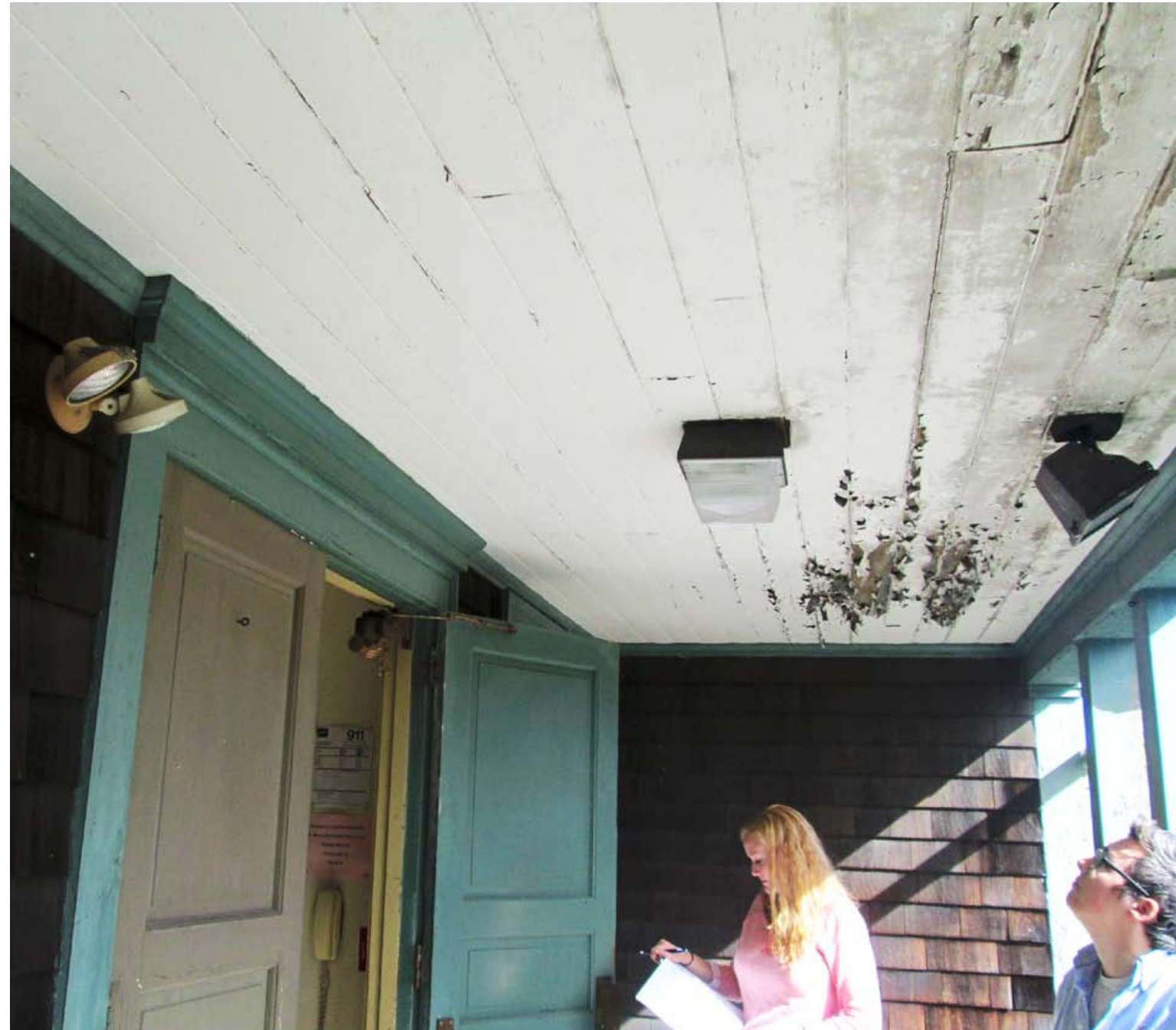
Students observe the parish house's front porch, a character-defining feature of the architectural style.
