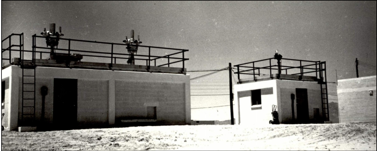
Figure 21. C-Station double and single cinetheodolite buildings, ca. 1951 (WSMR Museum Archives)
