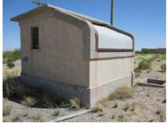
¾ view of the exterior, view northeast
