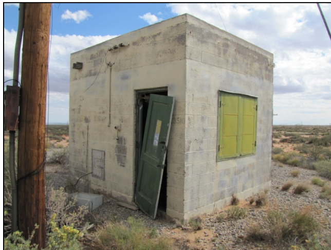
Figure 36. Camera Building, Tare Site, 2016
