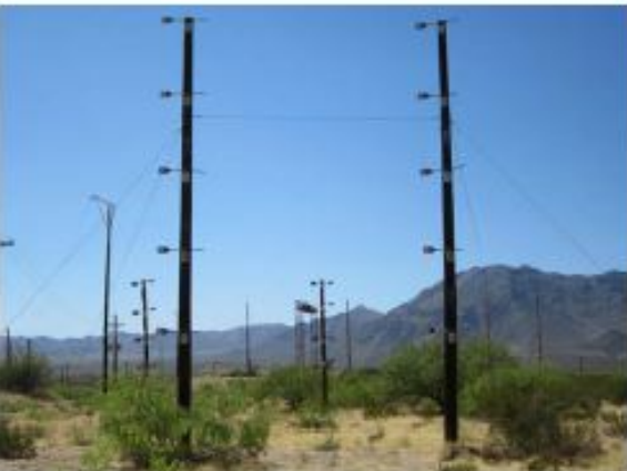
Overview of 4 calibration poles associated with building, view west
