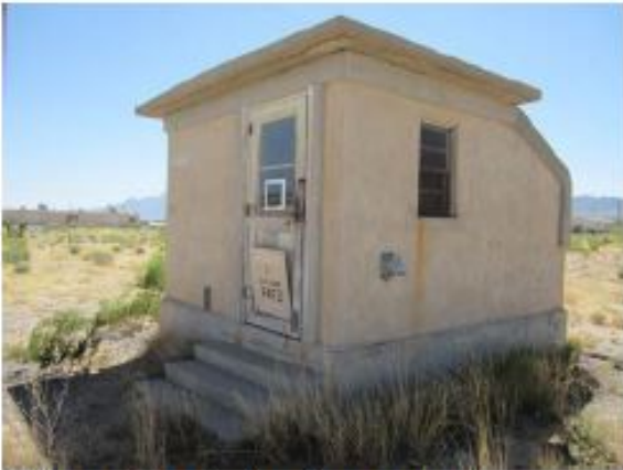
¾ view of the exterior, view southwest
