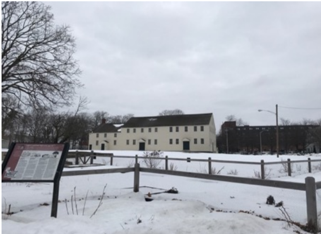
Figure 33: The Great Friends Meeting House as it stands today (21 Farewell Street), Photographed by: Arianna Marchetti, 11 Jan. 2018.
