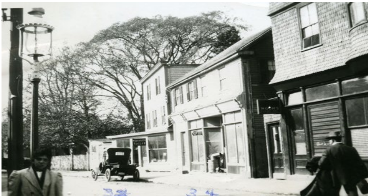
Figure 17: Mixed-use buildings on Marlborough Street - early 20th century. Courtesy of The Newport Historical Society.
