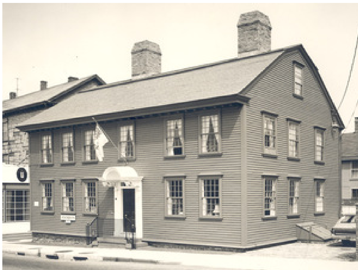
Figure 5: Photograph of the John Coddington House post restoration in the early 1970s. Courtesy of The Newport Historical Society.
