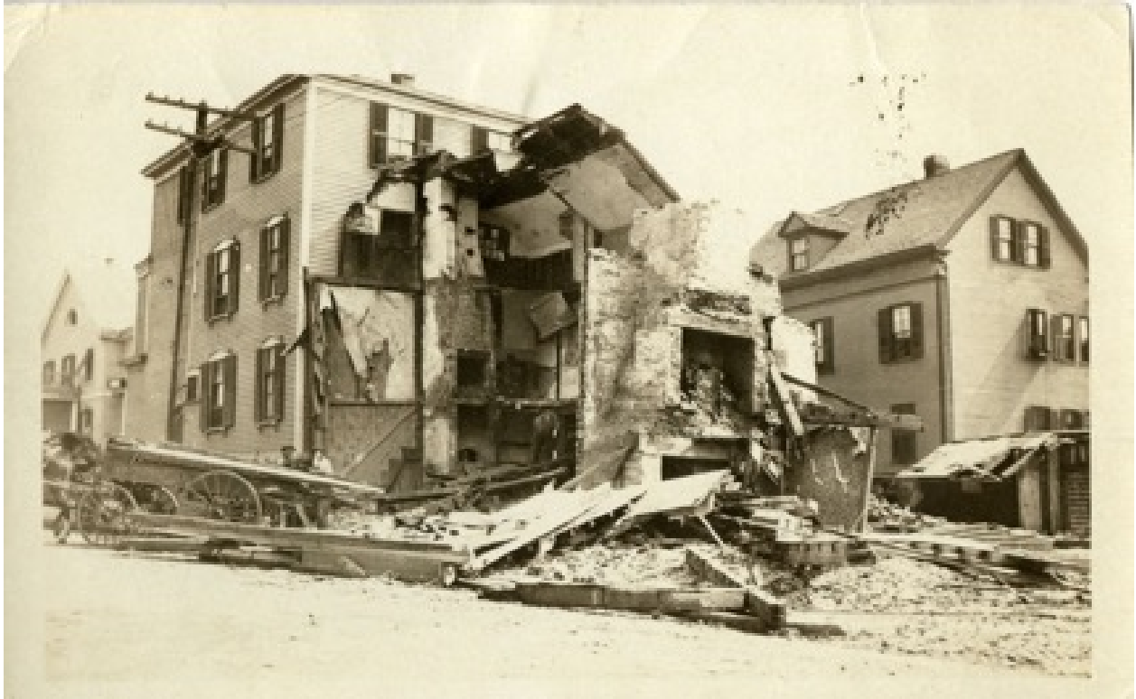
Figure 20: Historic home next to the Jailhouse on Marlborough Street undergoing demolition in the early 20th century. Courtesy of The Newport Historical Society.
