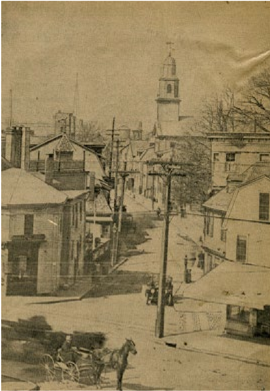
Figure 16: View of Marlborough Street from Broadway Street - early 20th century. Courtesy of The Newport Historical Society.
