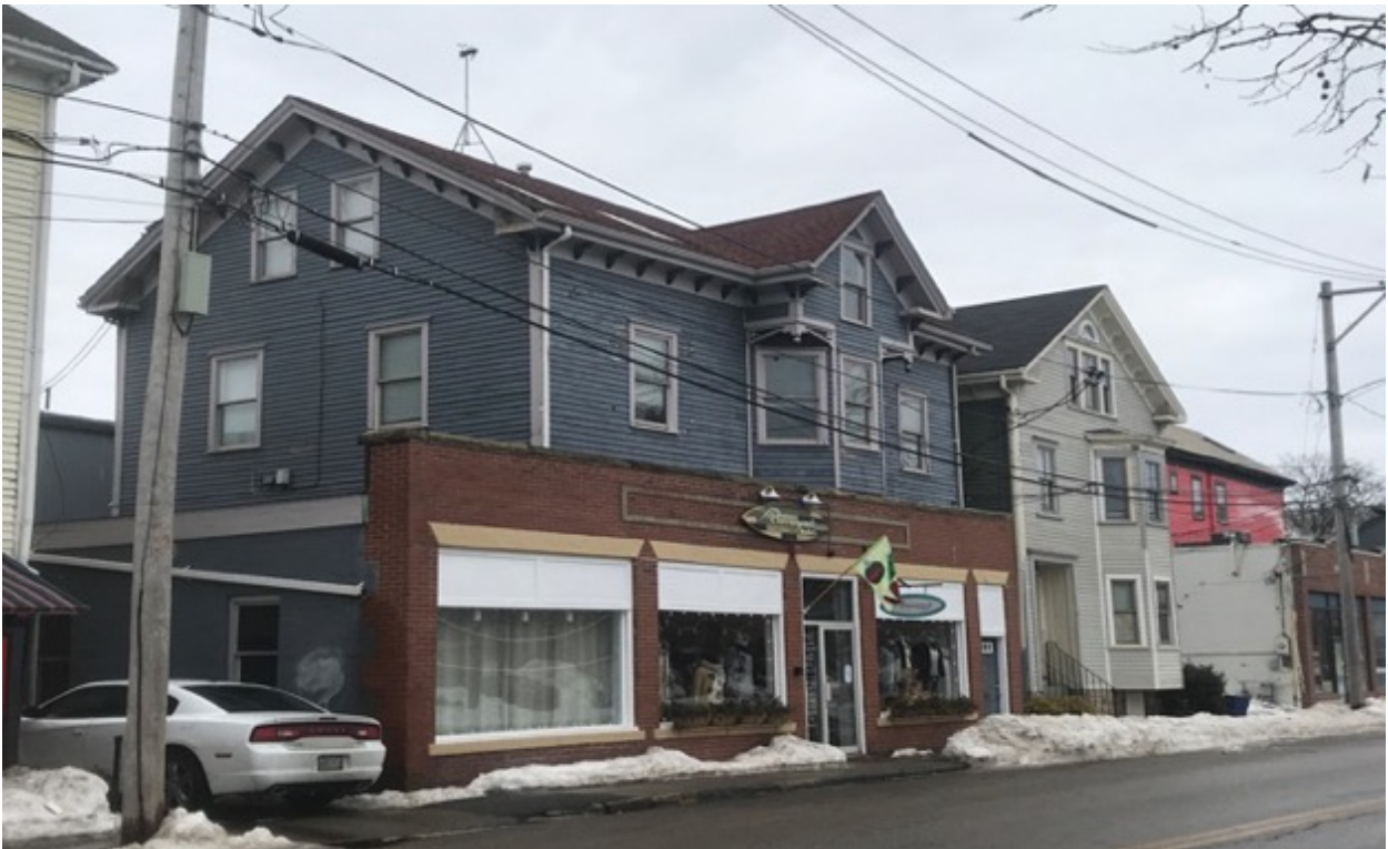
Figure 50: Example of twentieth century mixed-use structure on West Marlborough Street. Photographed by: Arianna Marchetti, 11 Jan. 2018.
