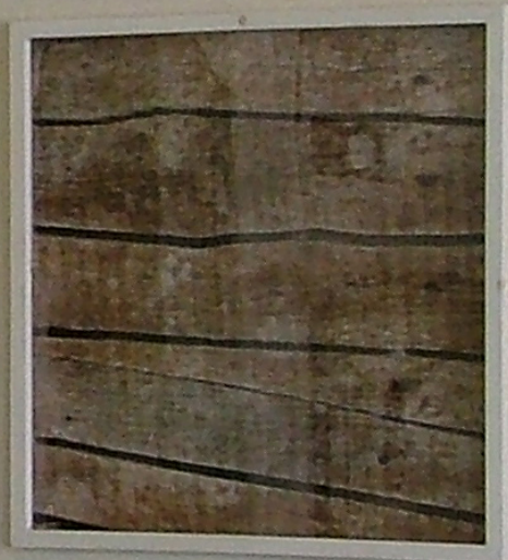
PLASTER HAS BEEN CUT AWAY TO REVEAL SPLIT BOARD LATH
