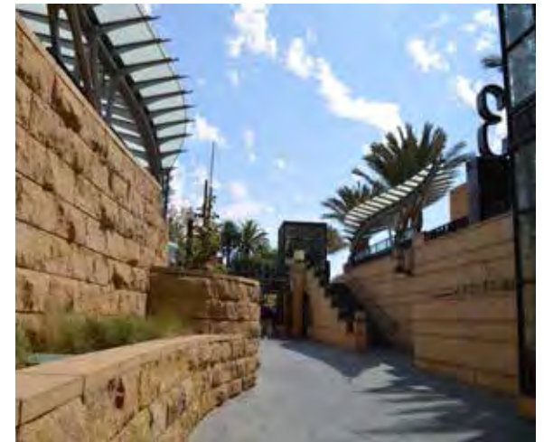
The below-ground portion of the Patsaouras Transit Plaza. This area connects directly with the East Portal. Access to the bus platforms is provided via elevators and stairs.
