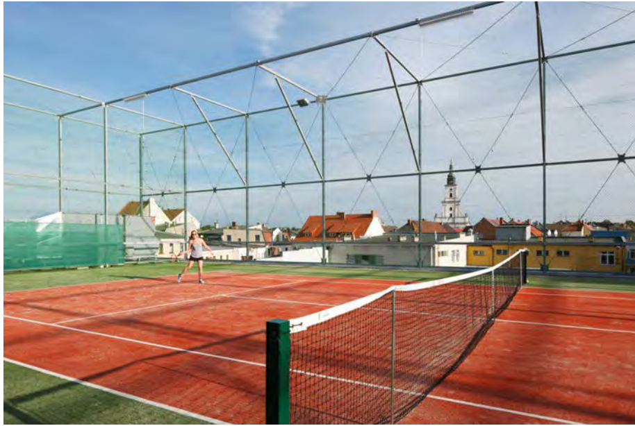
Tennis Courts on the roof
