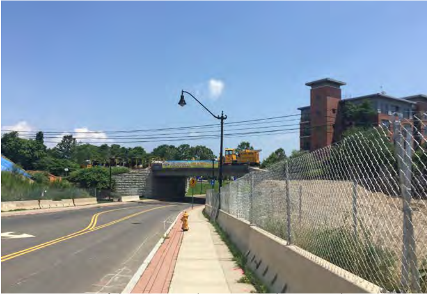
View of the train tracks crossing the street above
