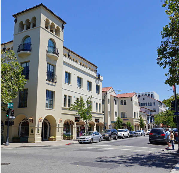
Commercial Building on Ramona Street
