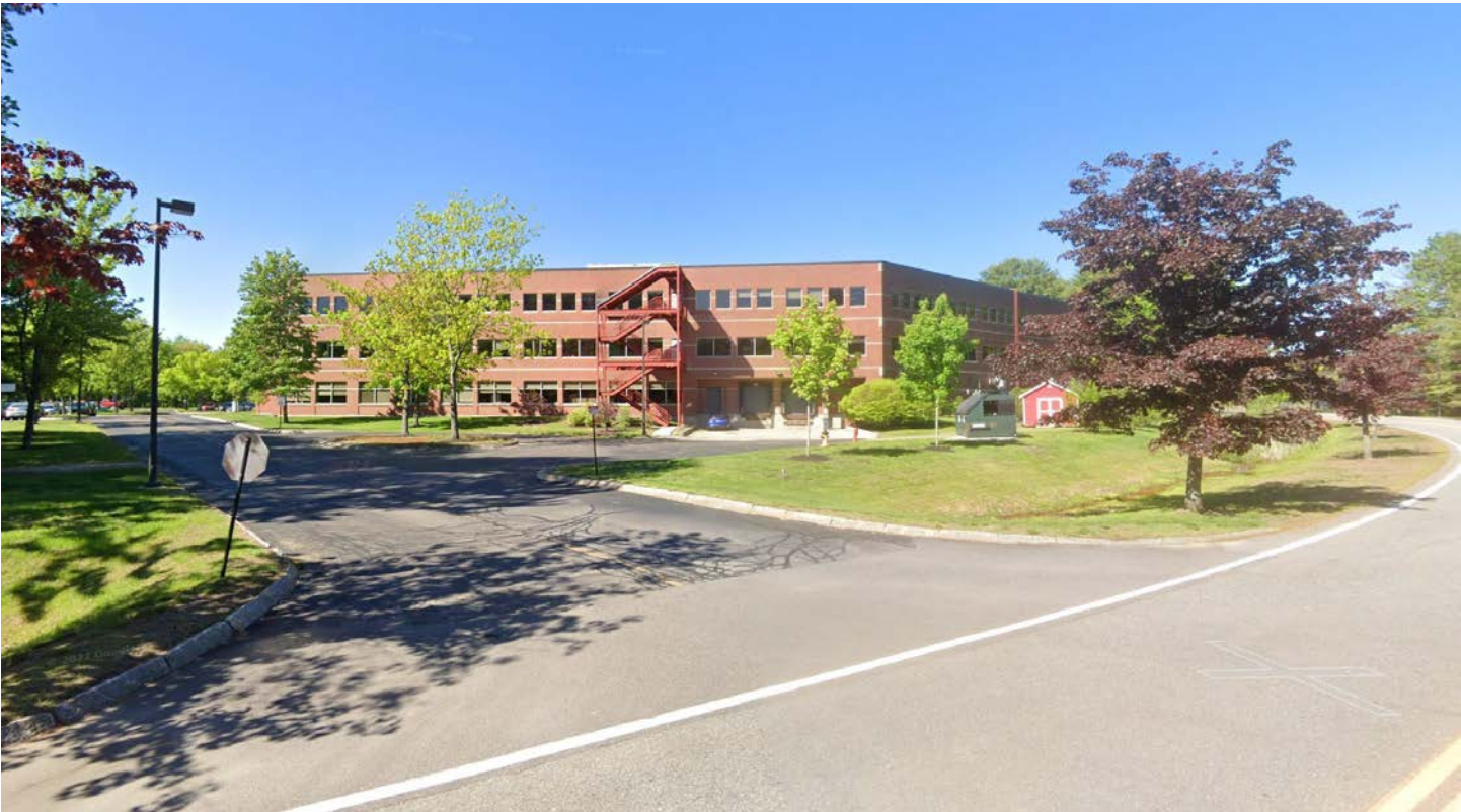
NORTHEAST ELEVATION SHOWING RETROFITTED EMERGENCY STAIR (FIGURE 17)
