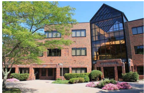
500 Southborough Drive (FIGURE 10)
