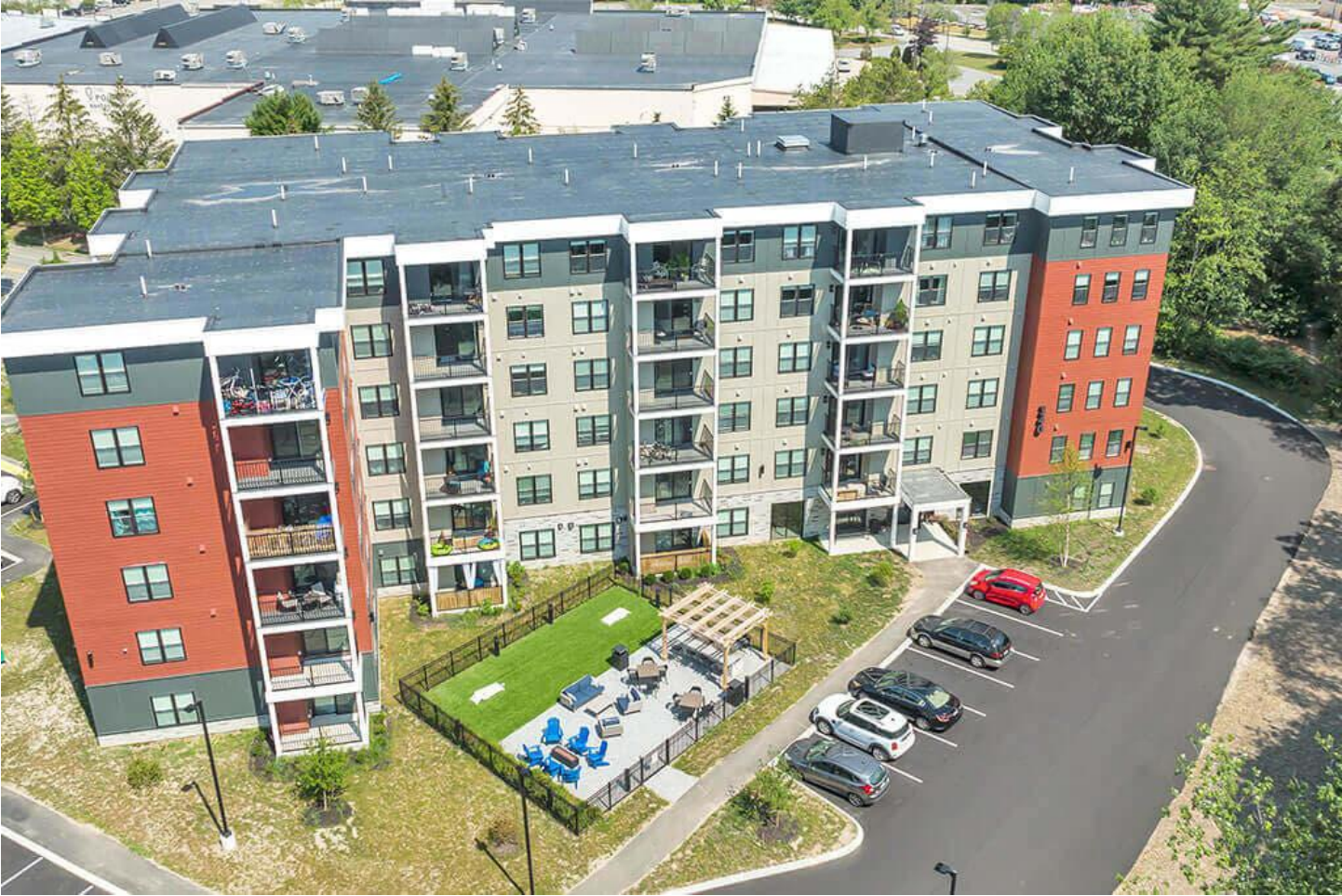
AERIAL VIEW OF BUILDING 340 (FIGURE 58)
