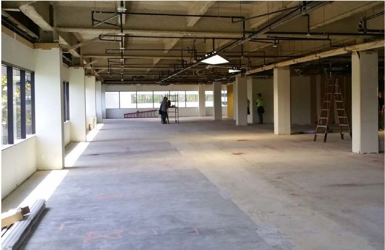
EXISTING STRUCTURE IMAGE (FIGURE 49)
