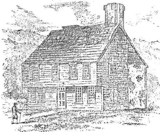
Governor William Coddington House, 1641. Demolished in 1835. From John Gorham Palfrey, History of New England , 1860, Vol. II, p. 62.
